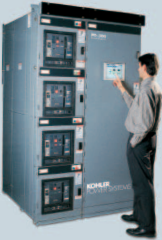
KOHLER PD-300 two-generator, two-feeder breaker, emergency standby system switchgear.
