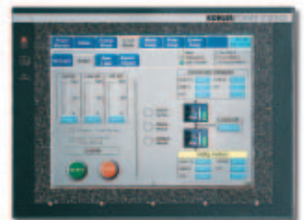
The latest Kohler PD-Series switchgear models replace switches and meters with an easy-to-use touch screen interface.
